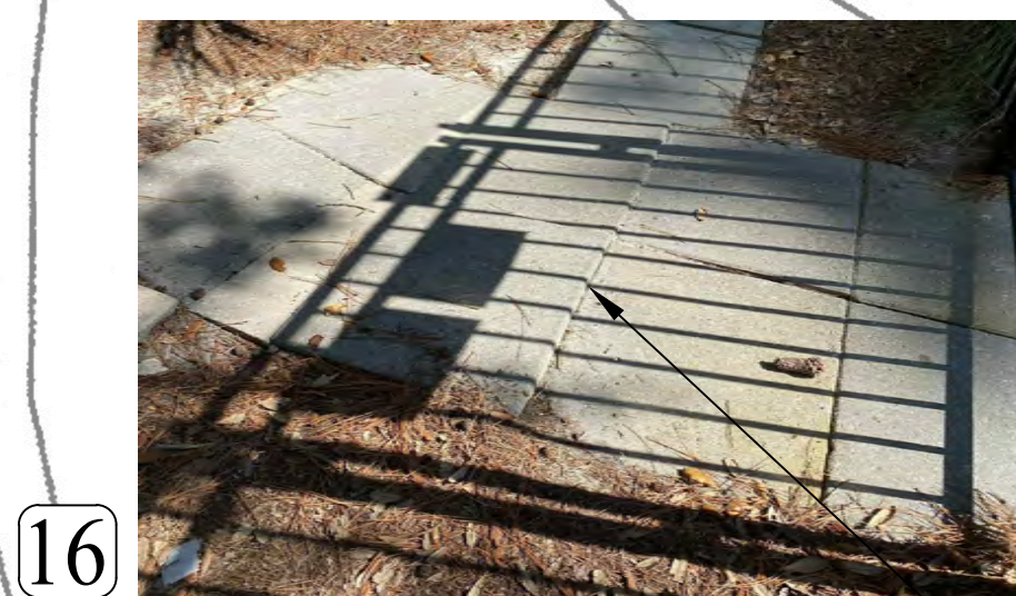
16 PROVIDE FORMAL PAVED ACCESS TO POOL, OR RESET STEPPING STONES FLUSH TO REDUCE TRIP HAZARD
