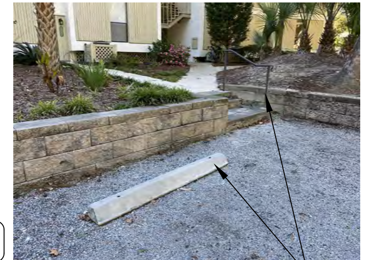
11 EXAMPLE OF WHEEL STOPS & HANDRAILS AT STAIRS
